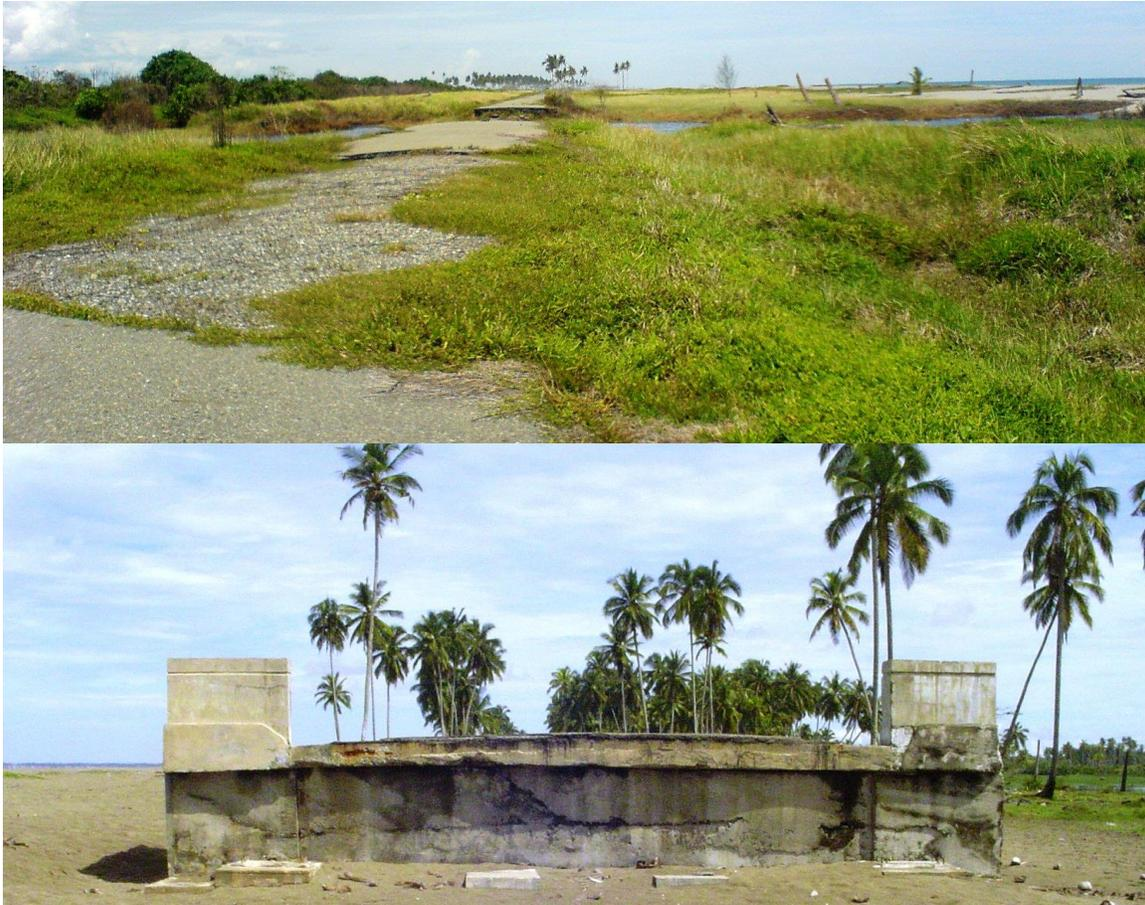
**Figure 1.4.** Damages to the coastal “national” road. Above: leftover asphalt and lacking bridge. Below: Road ends on a broken bridge over what before used to be a creek of small watery area. Close to the previously existing villages of Suak Ulue and Suak Sireen (Source: author).
