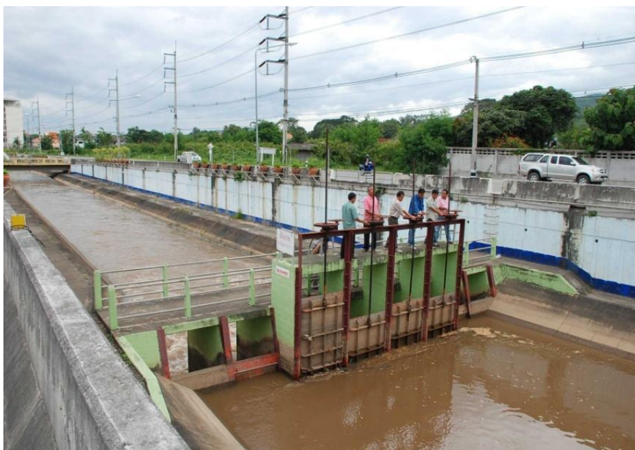
Figure 4.2: The IWUG leaders and MIP officers regulating water flow in the main canal
