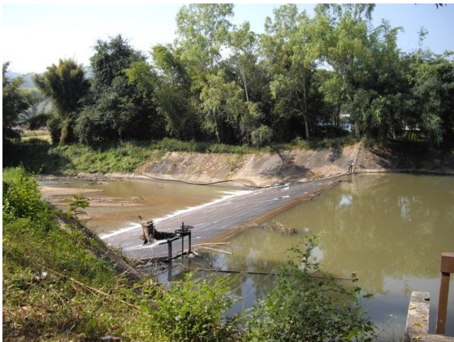
Figure 4.3: The weir of the Na Huek muang fai group located at the Mae Rim River
